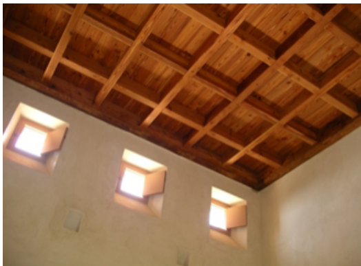
Ceiling Detail, Living Room
